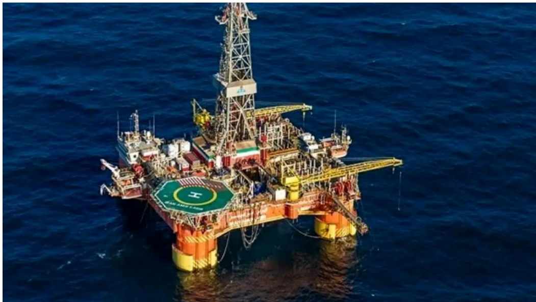
Fig. 1. The S1 wellhead platform in the Salman Oil Field
